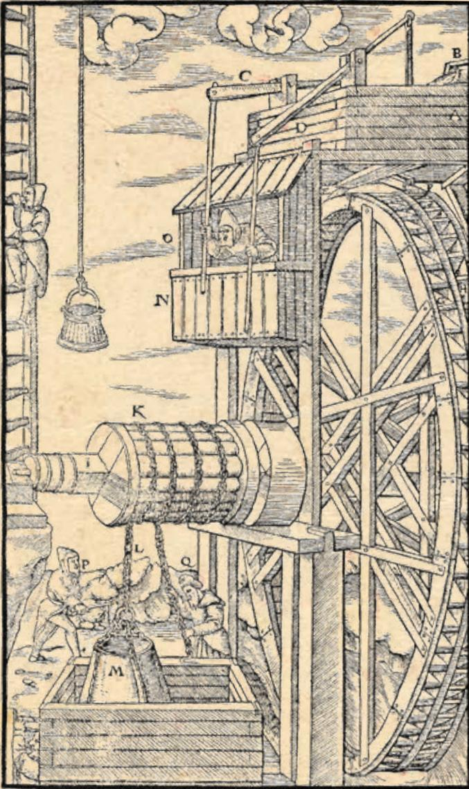
Water wheel powering a mine hoist. *De re metallica*, 1566
