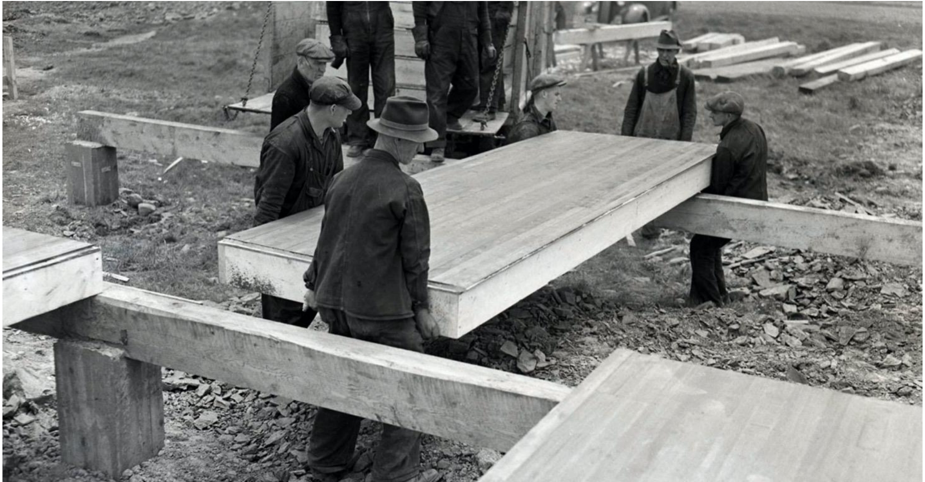
North and West-end Halifax house assembly of pre-fab panels. Public Archives of Nova Scotia, 1941
