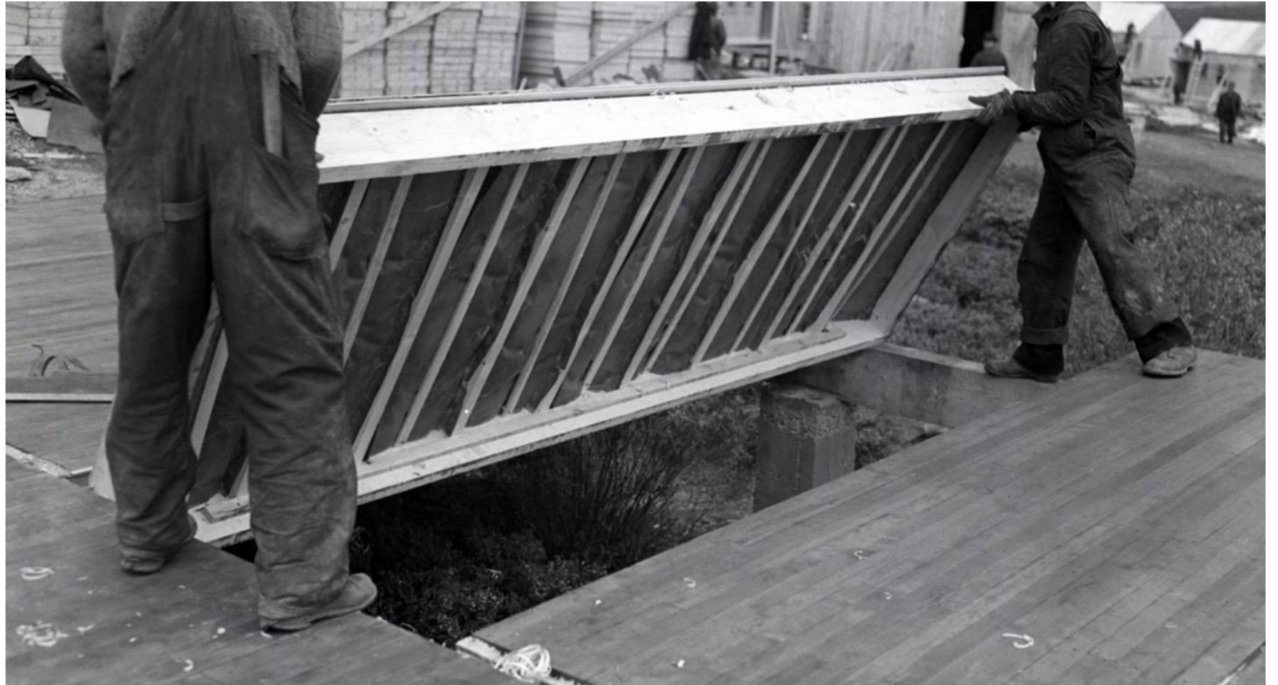
Floor panel installation (including finished hardwood). Public Archives of Nova Scotia, 1941
