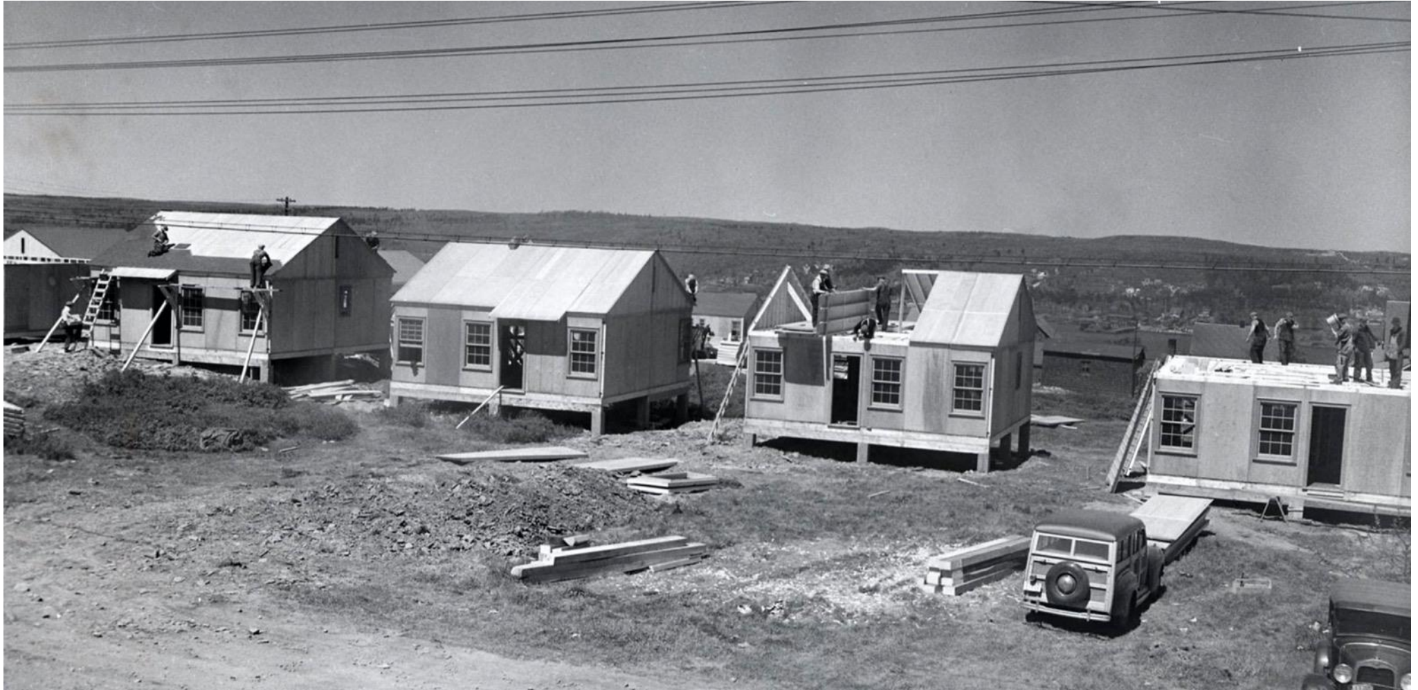
War-time Halifax house construction. Public Archives of Nova Scotia, 1941
