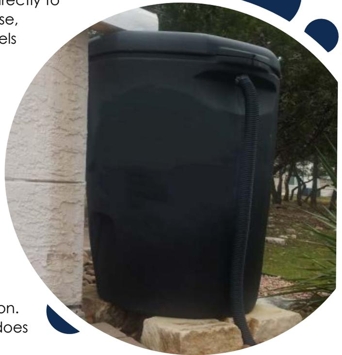
Elevating a rain barrel that have spouts at the bottom can make using the water easier by increasing the water pressure.
