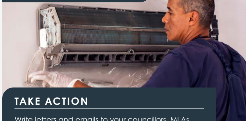
A worker doing cleaning work on a heat pump. PHOTO: Aleksej Sarifulin/iStock
