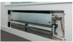
Figure 8.2 - Example of a Perimeter Fan Coil Unit Replacing a Radiator
