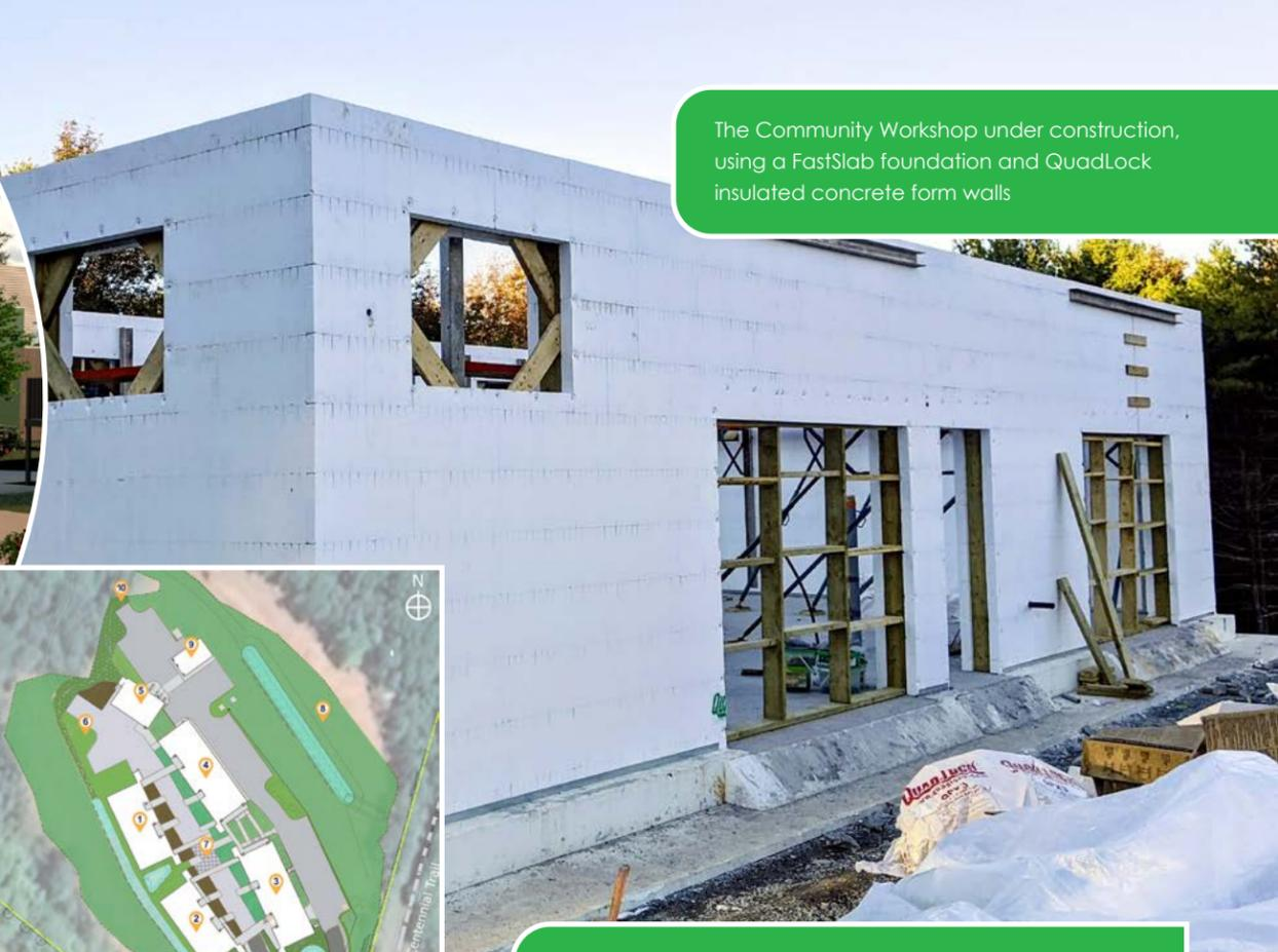
The Community Workshop under construction, using a FastSlab foundation and QuadLock insulated concrete form walls
